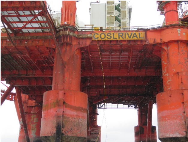
Fig. 5 – Photograph showing the rig COSL RIVAL
